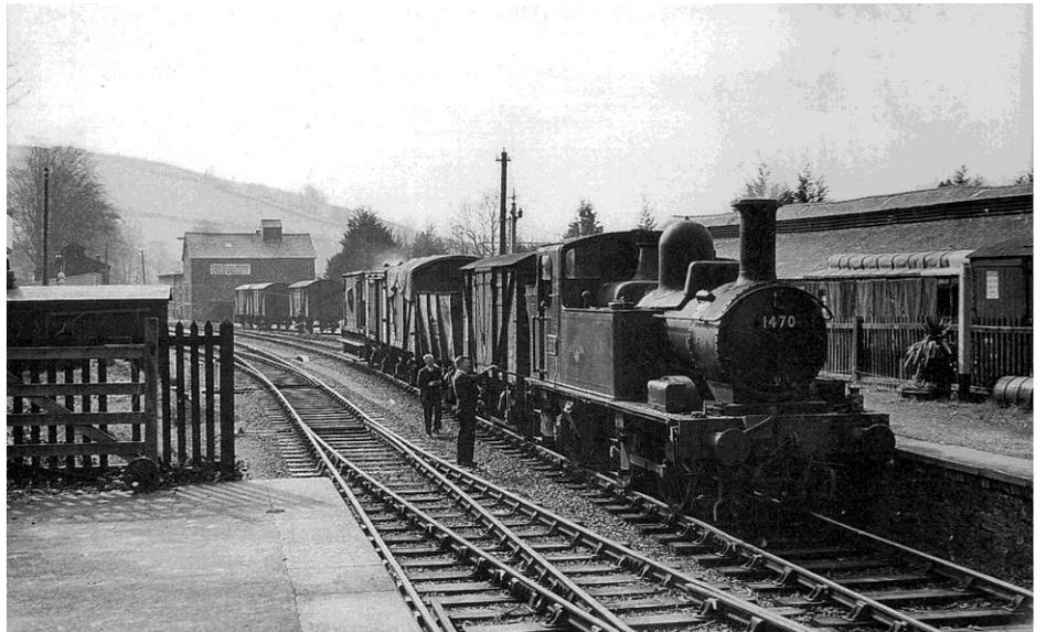
*The wire for the Up Starting Signal ran along the fence line. The wire can be seen attached to a fence post just above the lamp on the loco. By this time the signal arm had been removed and the wire was slack. Here 1470 is seen during the goods only period, by then in lined green livery with late logo and turned to run with chimney towards Ashburton. Photo: Alan Taylor Collection - [www.alextrack.co.uk](http://www.alextrack.co.uk)*
